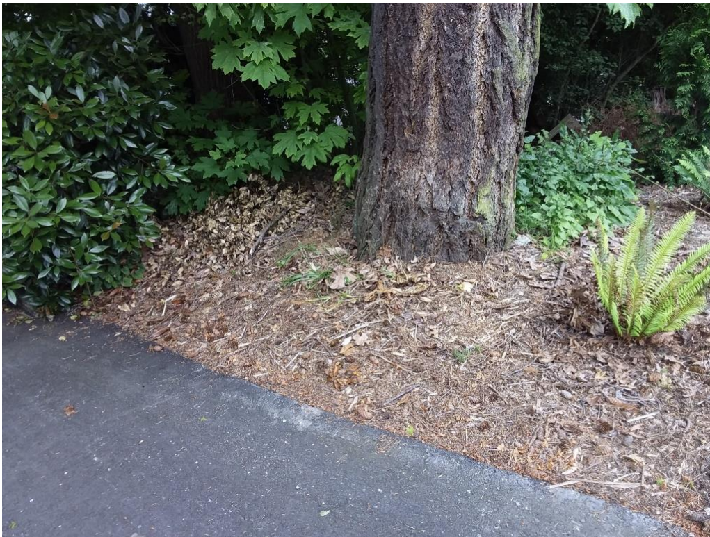
Figure 5. Photo of base of #2 fir showing malformation and proximity of the new pavement.
