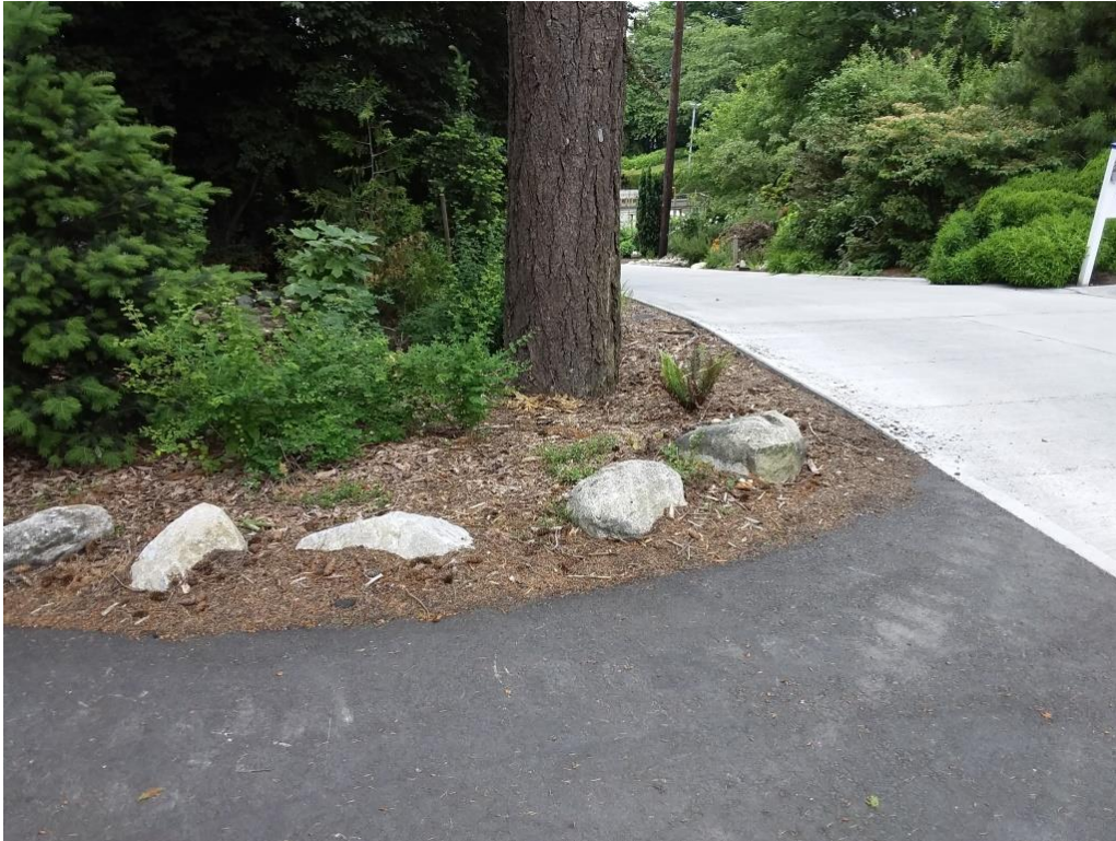
Figure 2. Photo of base of #1 fir showing repaving encroachment.
